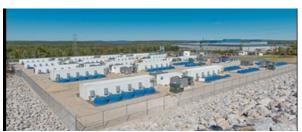
Figure 10 - Beacon FES Hazel, PA, 20 MW, Operating since Q3 2013
