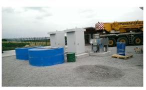
Figure 11: Two modular Beacon FES systems installed in Ireland for Schwungrad Energy as a renewable / battery hybrid demonstration.
